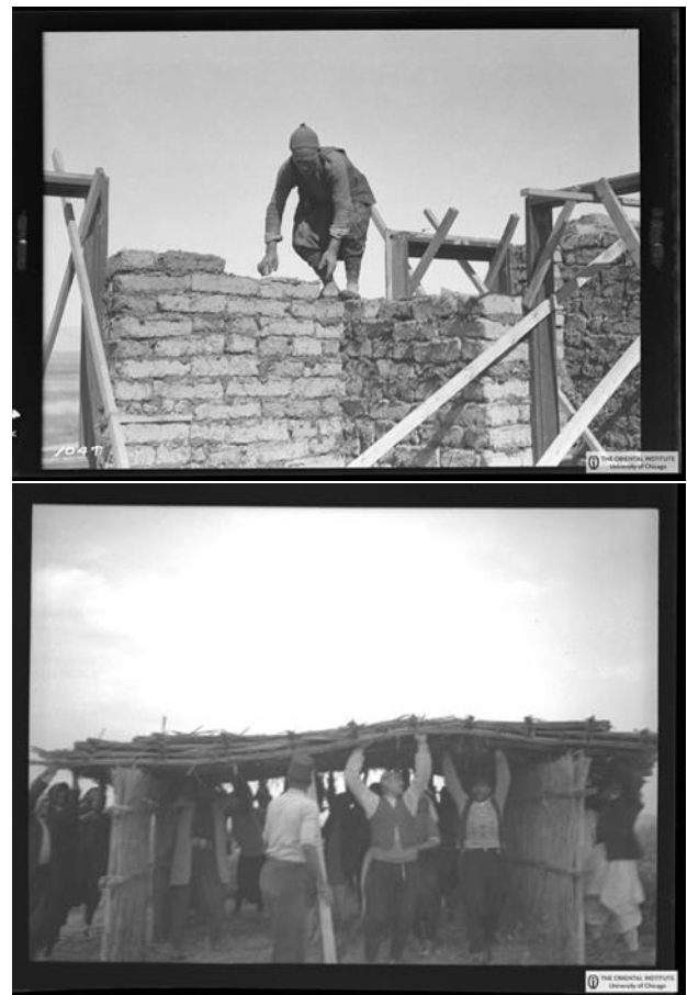
Figure 9a and 9b. Construction of the excavation house with mudbrick using an adaptation of traditional technologies (ISAC DPA Tayinat 104-T; top) and construction of a reed hut, which was later used as the ceramics workshop (ISAC DPA Tayinat 989-T; bottom). (Images: ISAC)
