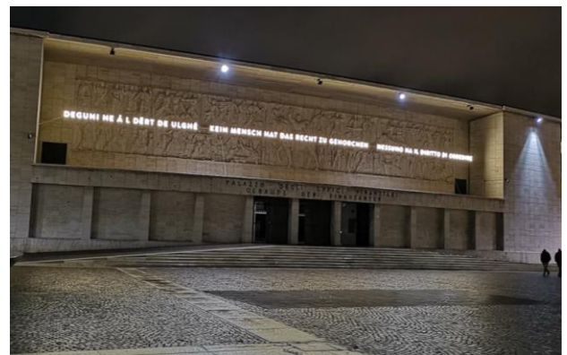
Figure 3. Facade of the former headquarters of the Fascist party in Bozen-Bolzano, now displaying a quote by Hannah Arendt (2018)
